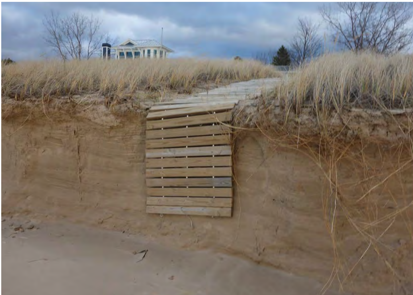
Grand Haven Beach Erosion.
